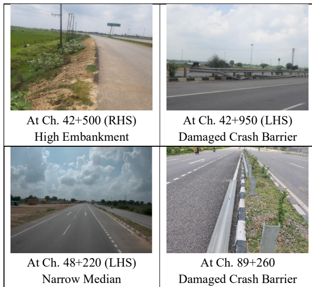
Figure 7 Photographs of High Embankment & Damaged Crash Barrier (NSV data)
